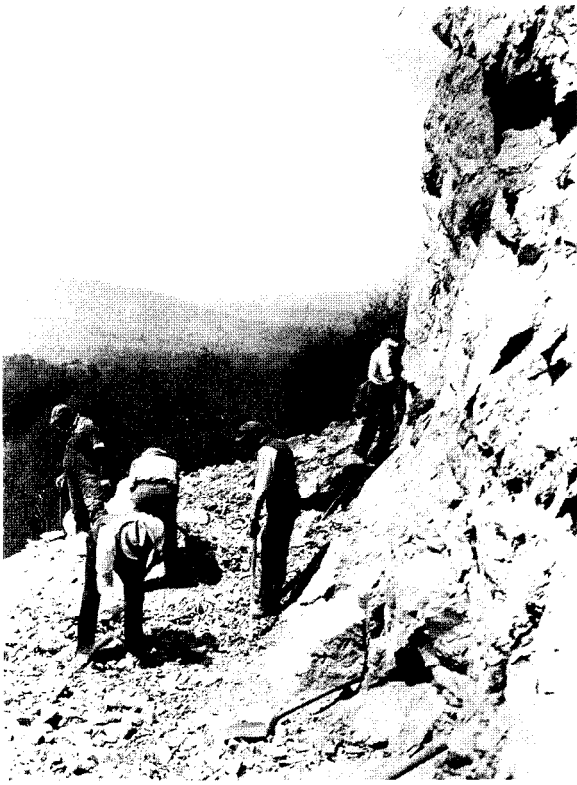
CCC road building, 1932
